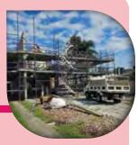
The second floor slab is poured, framing, structural steel, doors and windows installed.
