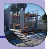
The foundations and ground floor slab are poured.
